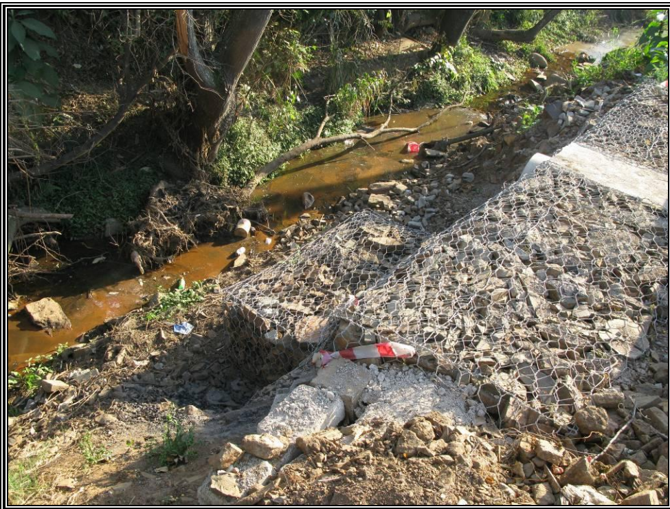
Photograph 2. Drainage line on the study property. Note the abundance of garbage.
