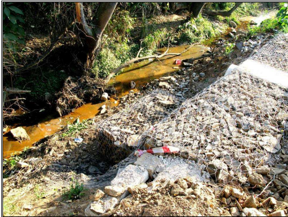
Photograph 1. Mkondeni Stream in an industrial area. Note the accumulation of solid wastes in the channel as well as evidence of oil or other such contaminants on the water. The channel is being scoured.
