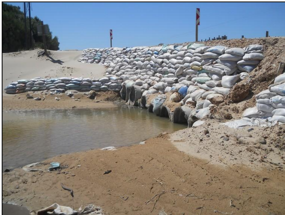
Figure 2: View of the temporary structure that is currently in place along the deviation allowing flow in the Sand River.
