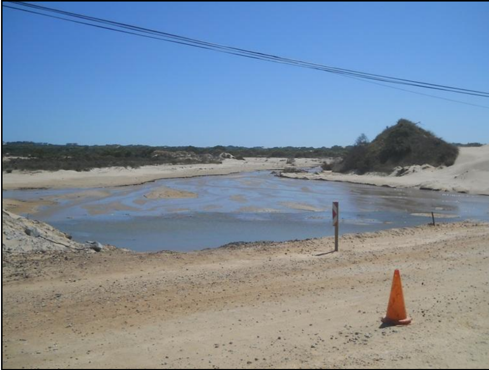
Figure 5: Upstream view of Sand River crossing.
