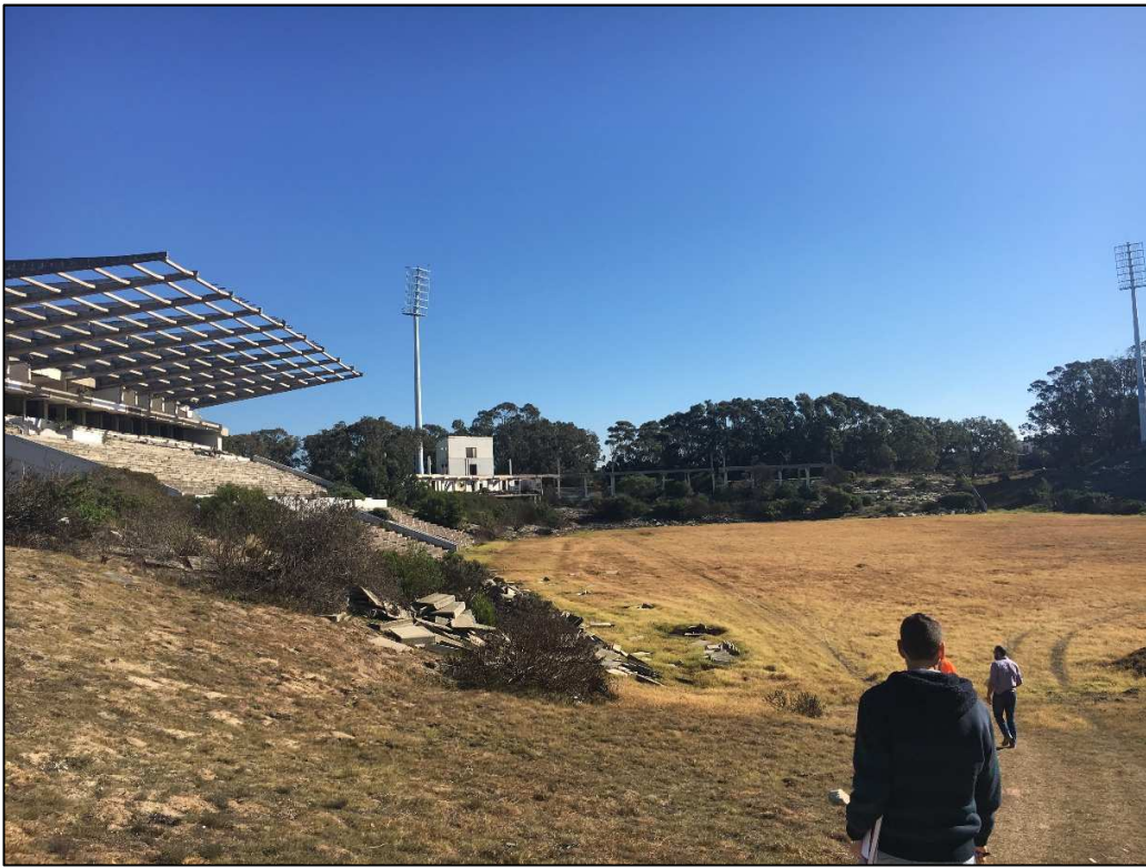
Photo 3: View of the corporate suites, located on the western side of the stadium facility.
